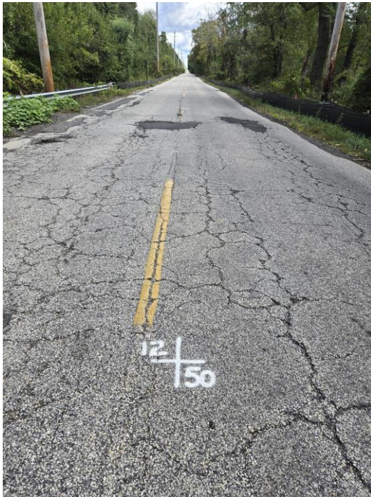
Figures 5 & 6 - Noon-Mathis Associates performs layout for full depth reclamation (FDR) segment.
