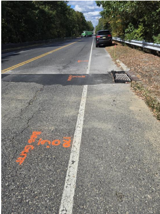
Figures 3 & 4 - Noon-Mathis Associates continues survey layout for concrete curb and concrete gutter.
