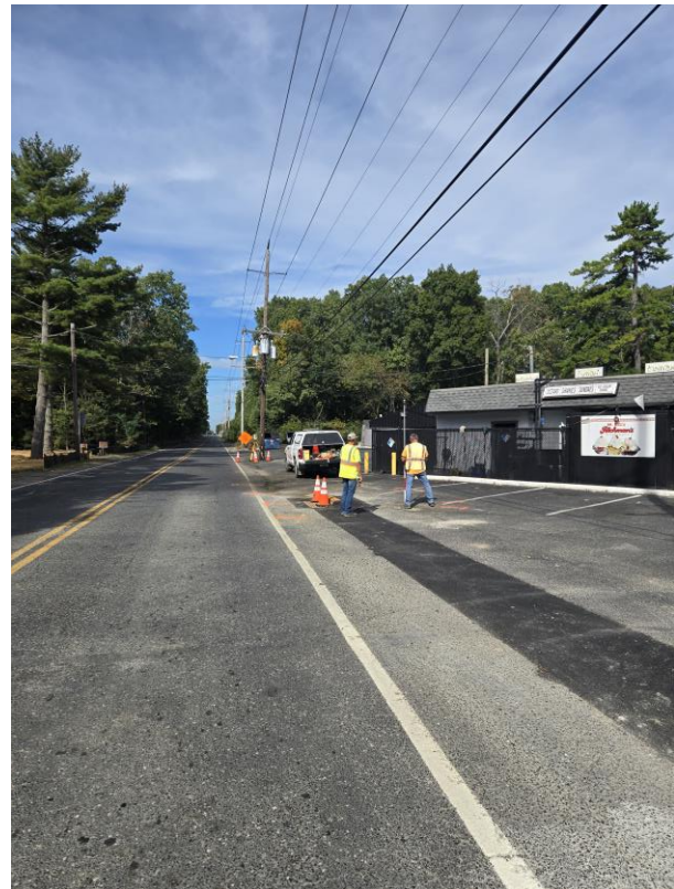
Figures 1 & 2 – Noon-Mathis Associates performing survey layout work for the installation of concrete curb and concrete gutter on West Fleming Pike (CR 723), Camden County.
