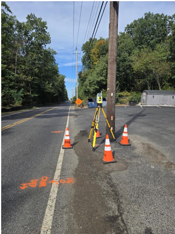
Figures 1 & 2 – Noon-Mathis Associates performing survey layout work for the installation of concrete curb and concrete gutter on West Fleming Pike (CR 723), Camden County.
