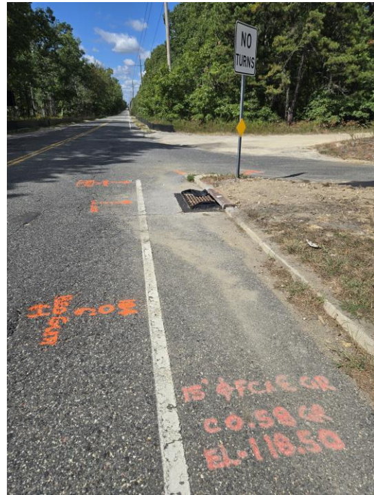
Figures 3 & 4 - Noon-Mathis Associates continues survey layout for concrete curb and concrete gutter.
