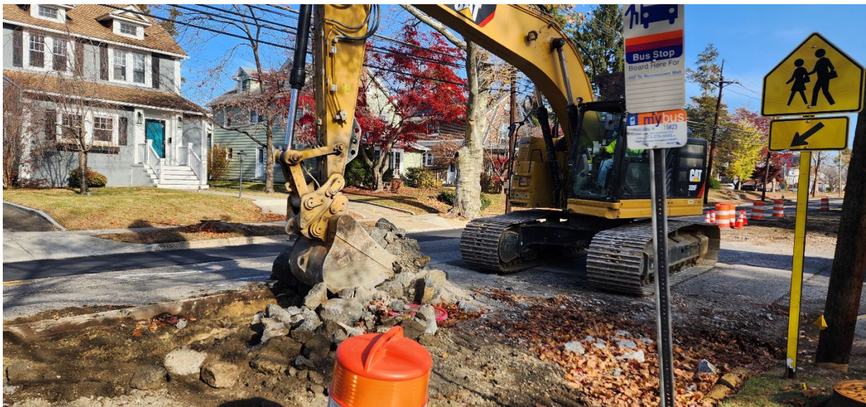
Figure 3: Continued removal of rubblized concrete pavement along eastbound lane
