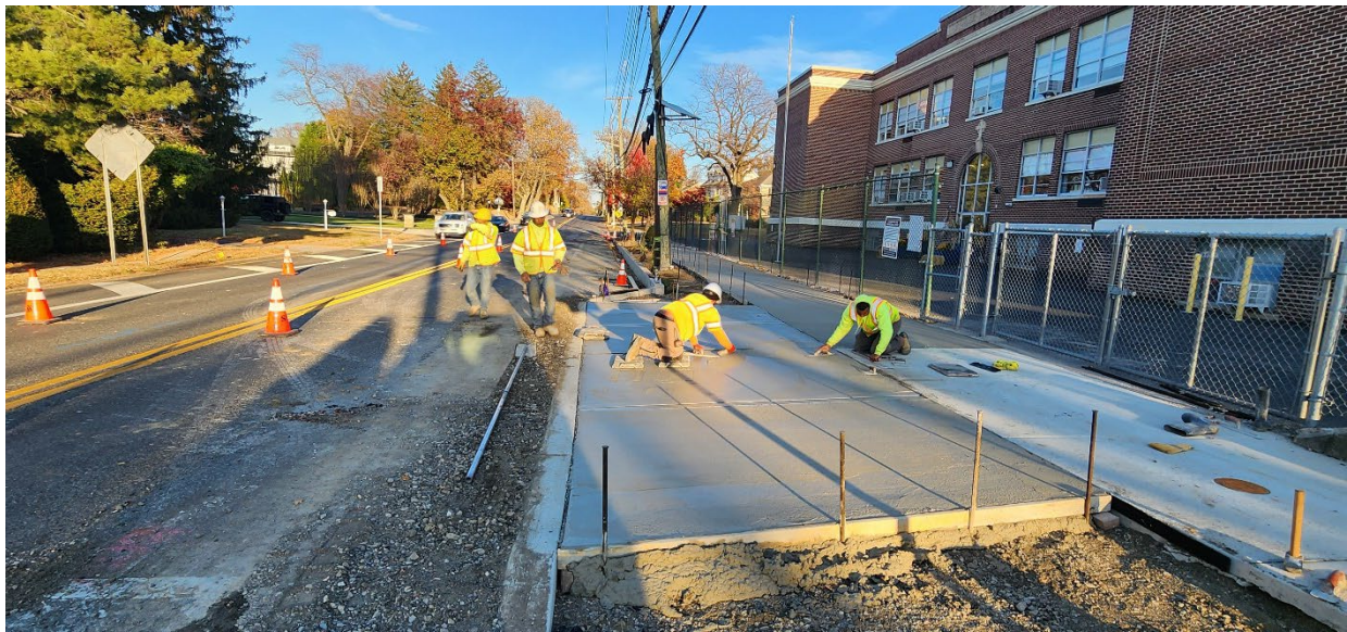
Figure:1 Installed sidewalks and ramps at Saint rose school
