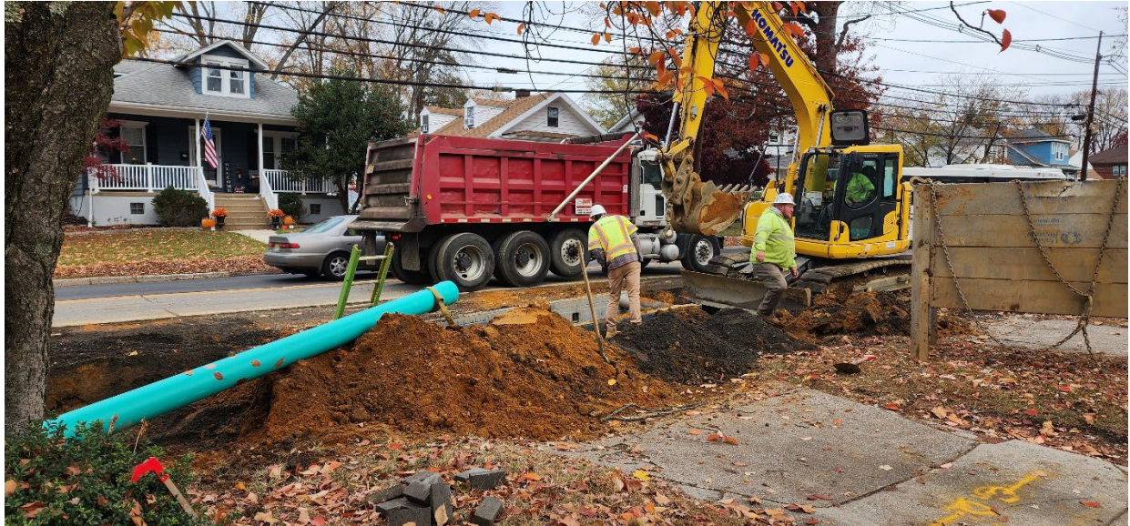
Figure 2: Continued sewer main replacement along Eastbound lane
