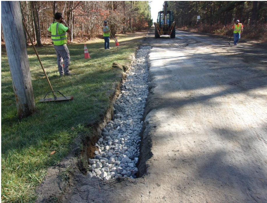
Figure 2 Repair to Soft Spot
