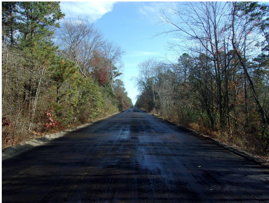
Figure 3 Tack Coat prior to Paving
