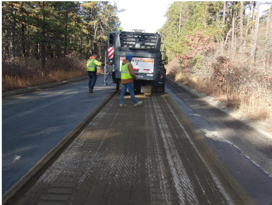
Figure 1 Mill to Subbase
