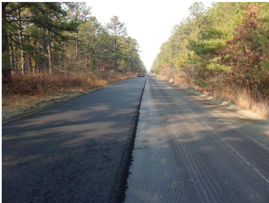
Figure 4 Paving for Phase 2
