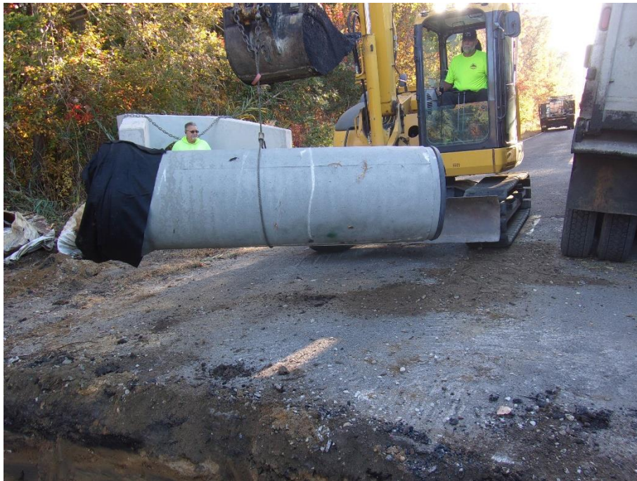
Figure 1 Continued Pipe Replacement (STA 83+50±)
