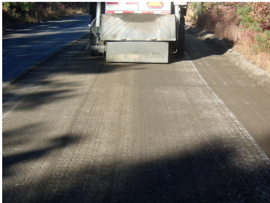
Figure 3 Start to Mill to Subbase (STA 12+00± to 82+00±)
