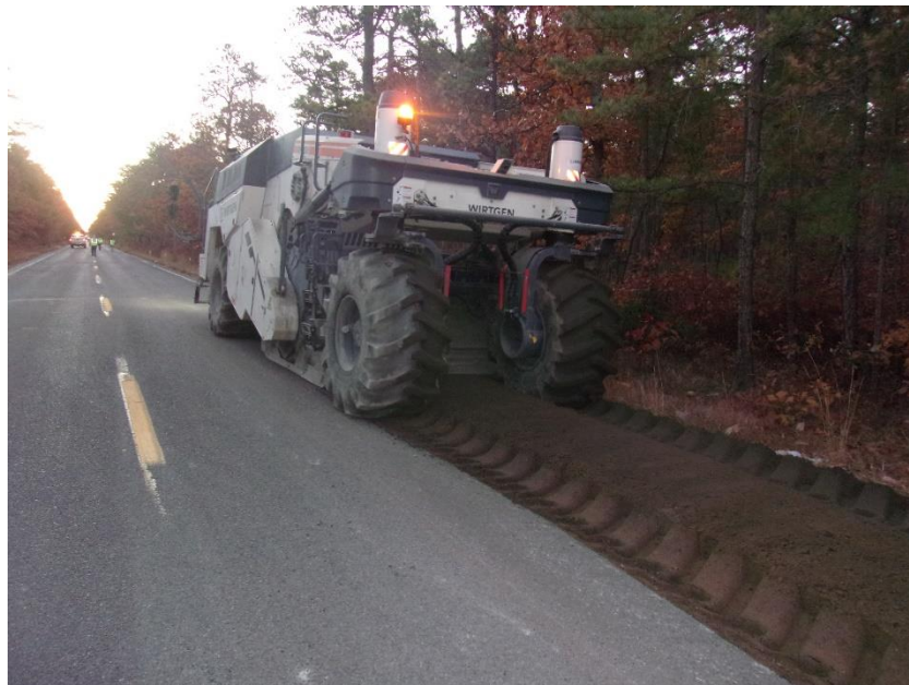
Figure 5 FDR Begins for Phase 2 at STA 82+25±
