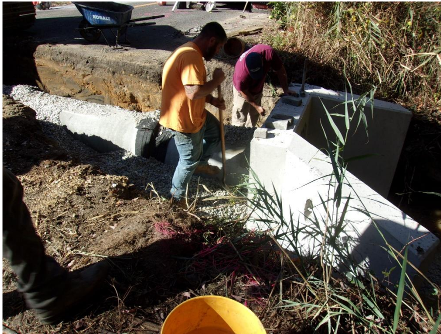
Figure 2 New Headwall Set at Storm Crossing (STA 83+50±)
