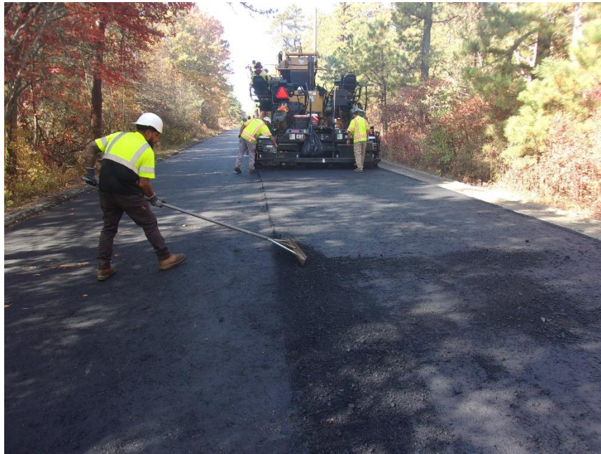
Figure 4 Phase 1 Base Pave (STA 12+00± to 82+00±)
