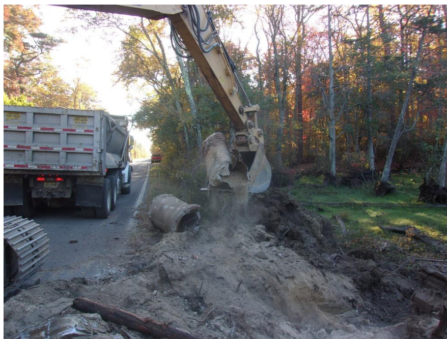
Figure 4 Removal and disposal of existing storm pipe (STA 83+50)
