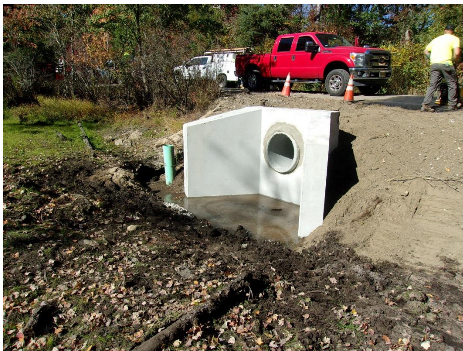
Figure 5 One (1) headwall and three (3) 8' pieces of 24" RCP installed (STA 83+50)
