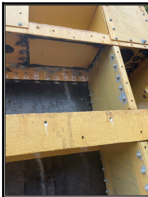
Figure 3: Replacement of Rivets.
