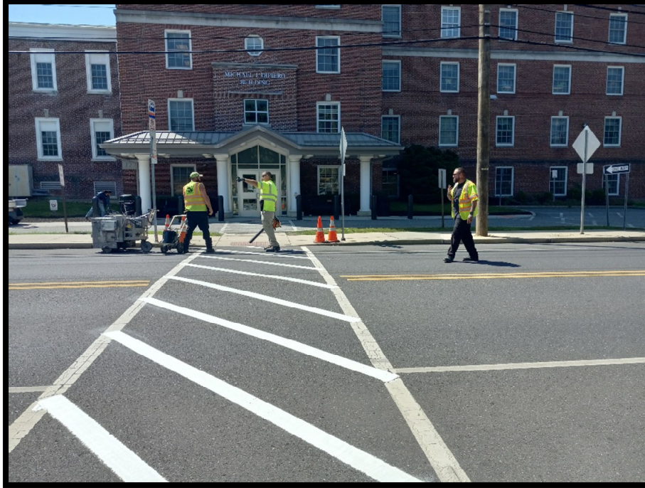
Photograph 4 – Typical Zebra Cross Walk striping being installed on Lakeland Avenue (CR 747).
