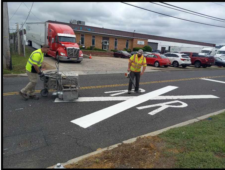
Photograph 4 – Typical Railroad Crossing Symbols being installed on Sherman Avenue (CR 760).
