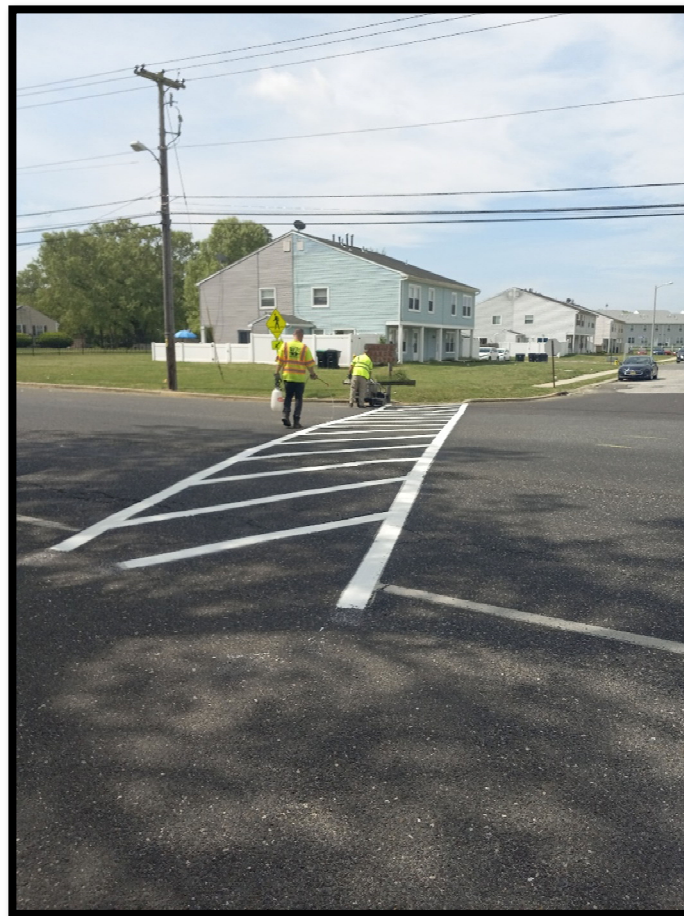
Photograph 1 – Typical Zebra Cross Walk Striping being installed.
