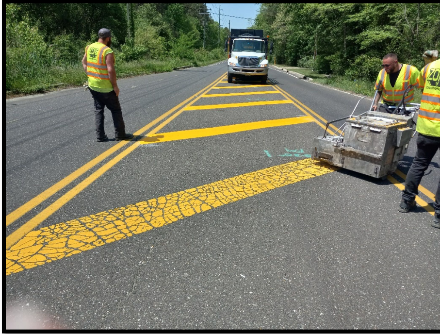
Photograph 2 - Typical 24" Yellow Thermoplastic Gore Striping being installed.
