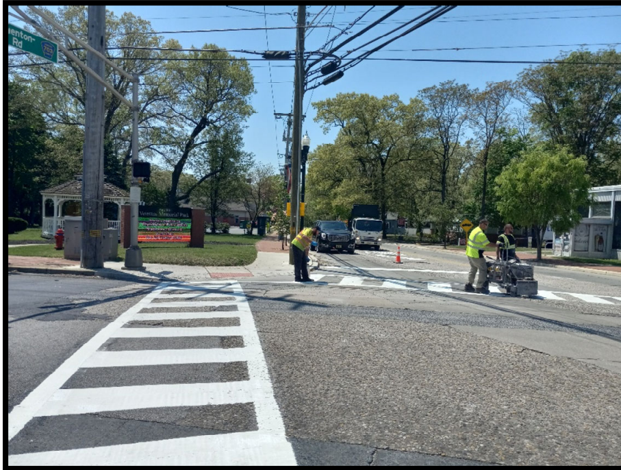
Photograph 4 – Typical Ladder Cross Walk being installed on Clementon-Erial Road (CR 703).
