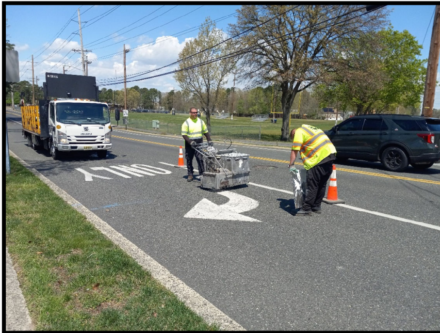
Photograph 3 – Arrows and “ONLY” being installed on Egg Harbor Road (CR 702).
