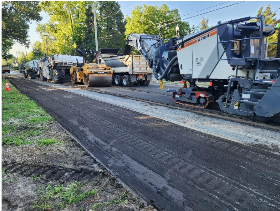
Figure 1. FDR Pulverization and Milling process
