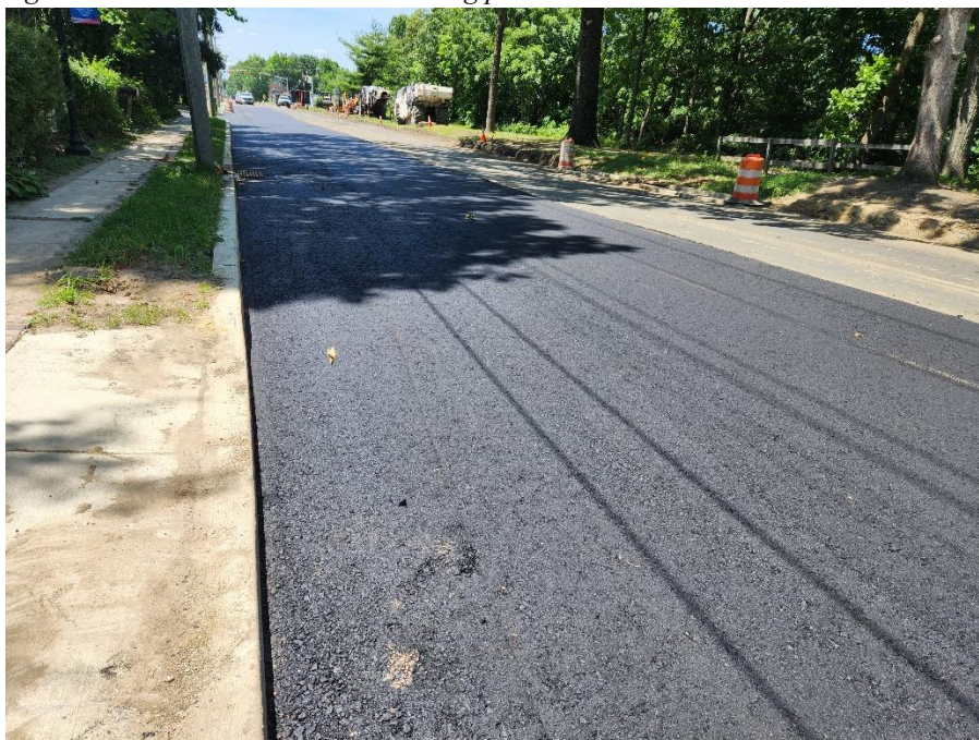
Figure 2. Base asphalt pavement along Berlin Road
