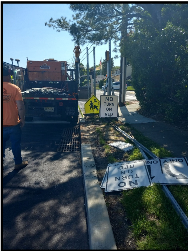
Photograph 1 – Sign installation subcontractor installing various Regulatory and Warning Signs.
