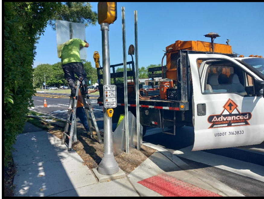
Photograph 3 – Sign installation subcontractor installing various Regulatory and Warning Signs.
