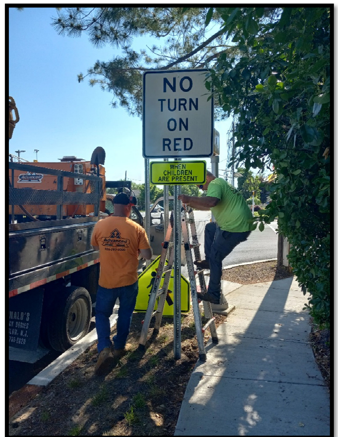
Photograph 2 – Sign installation subcontractor installing various Regulatory and Warning Signs.
