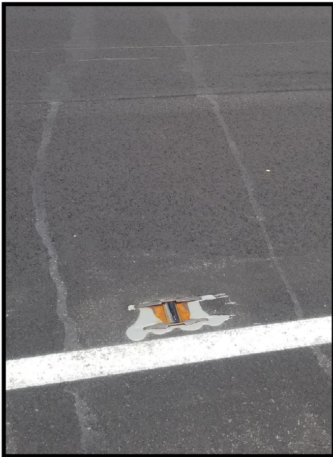
Photograph 1 – Raised Pavement Marker installed along Greentree Road.
