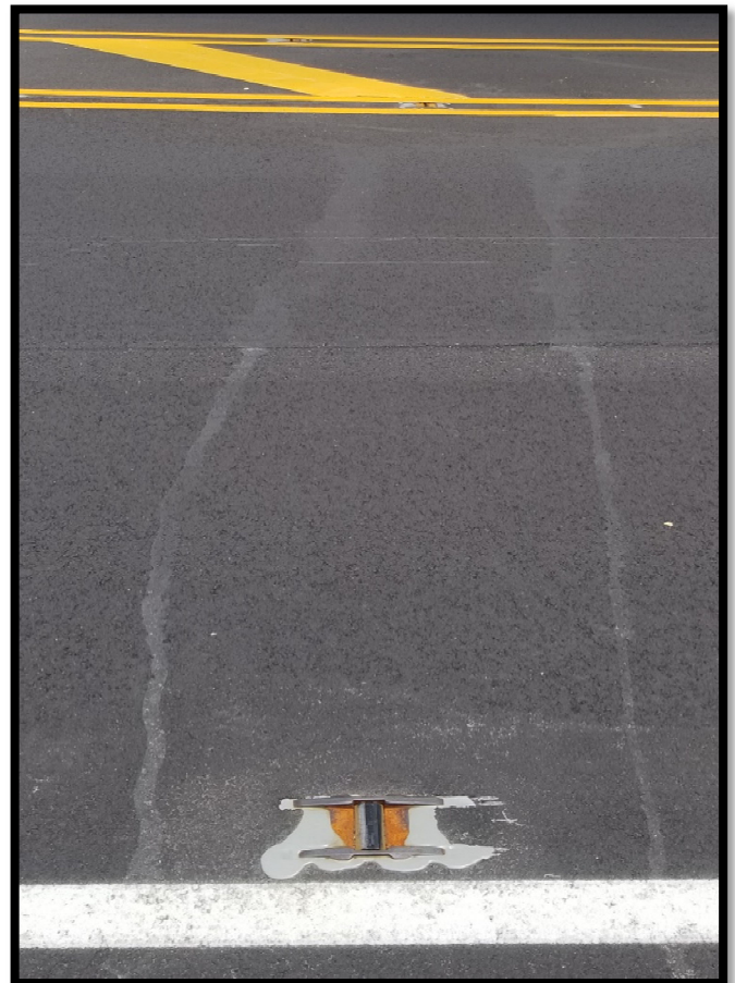
Photograph 2 – Raised Pavement Markers installed along Greentree Road.
