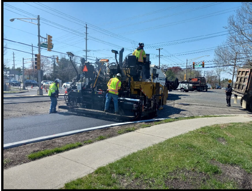
Photograph 6 – Hot Mix Asphalt Surface Course being installed near Springdale Road.
