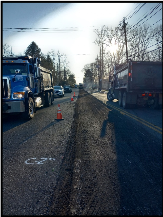
Photograph 1 – First pass with milling machine.
