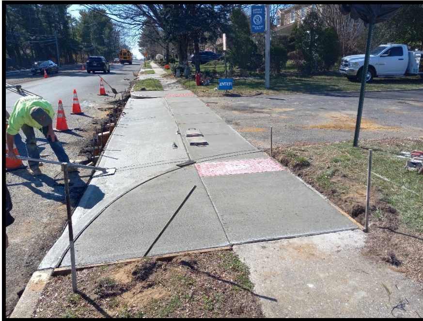
Photograph 5 – Concrete apron being installed in front of Cooper Elementary School.
