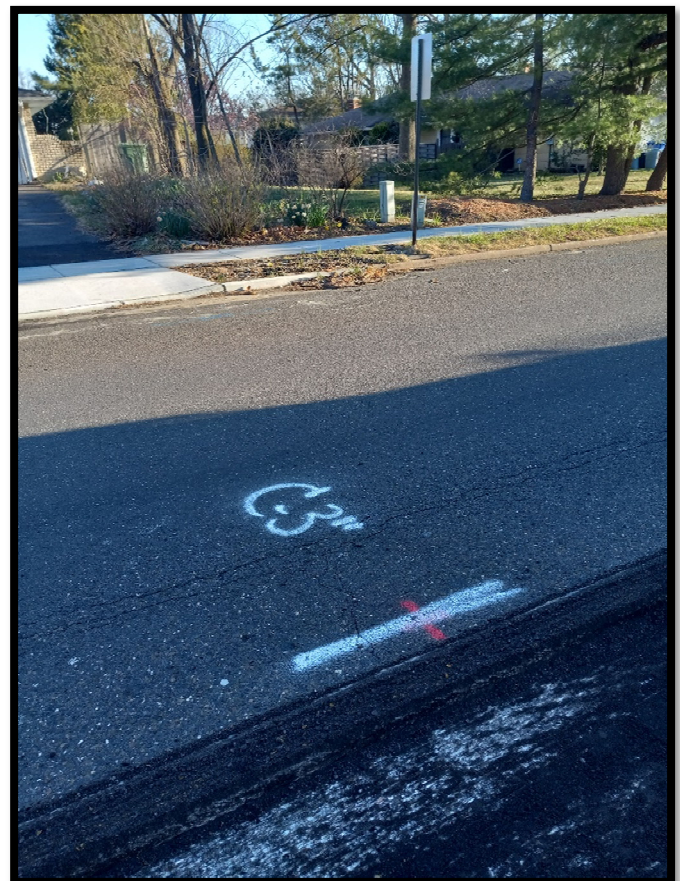
Photograph 2 – Area of mill with 3" cut.
