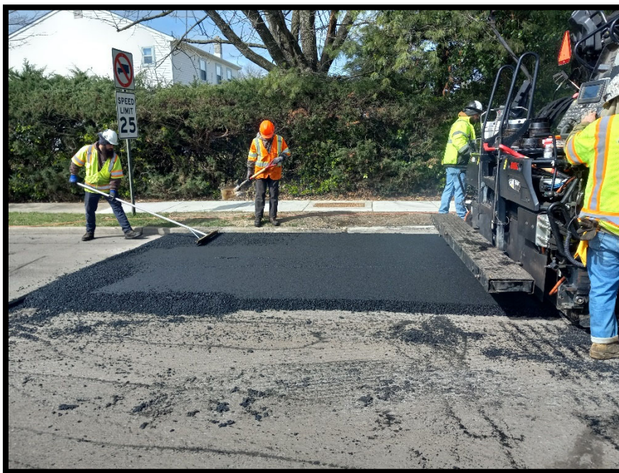
Photograph 6 – Hot Mix Asphalt Surface Course being installed.
