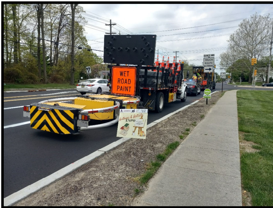
Photograph 6 – Subcontractor installing traffic striping and markings.
