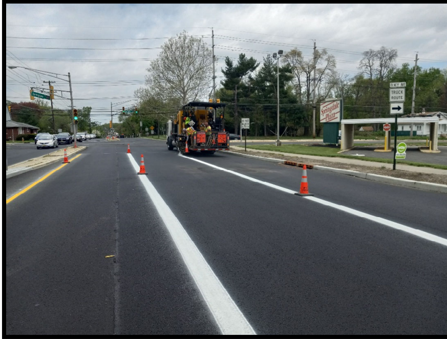
Photograph 7 – Subcontractor installing traffic striping and markings.
