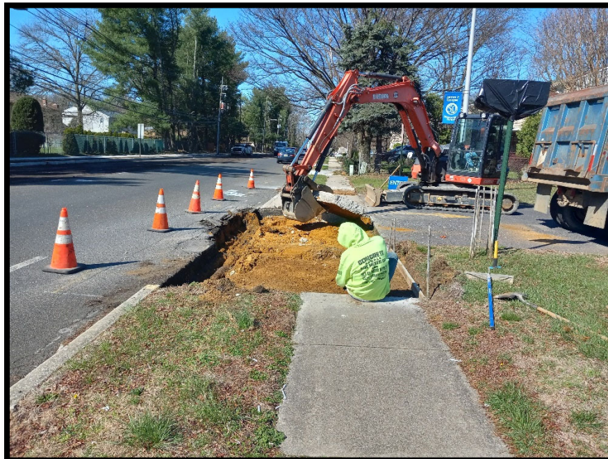
Photograph 4 – Concrete apron being replaced in front of Cooper Elementary School.
