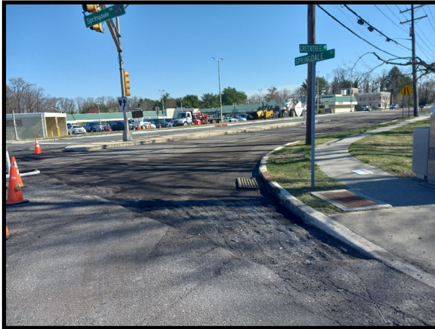
Photograph 3 – Milling complete at Springdale Road intersection.
