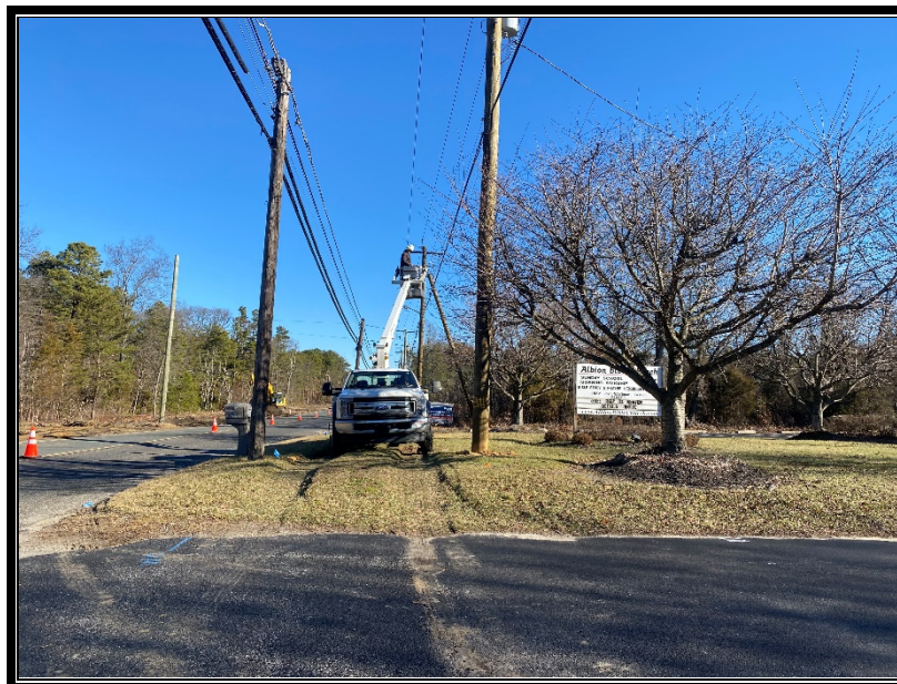
Figure 3: Comcast's sub-contractor Urban Cable relocating cable to new utility poles.
