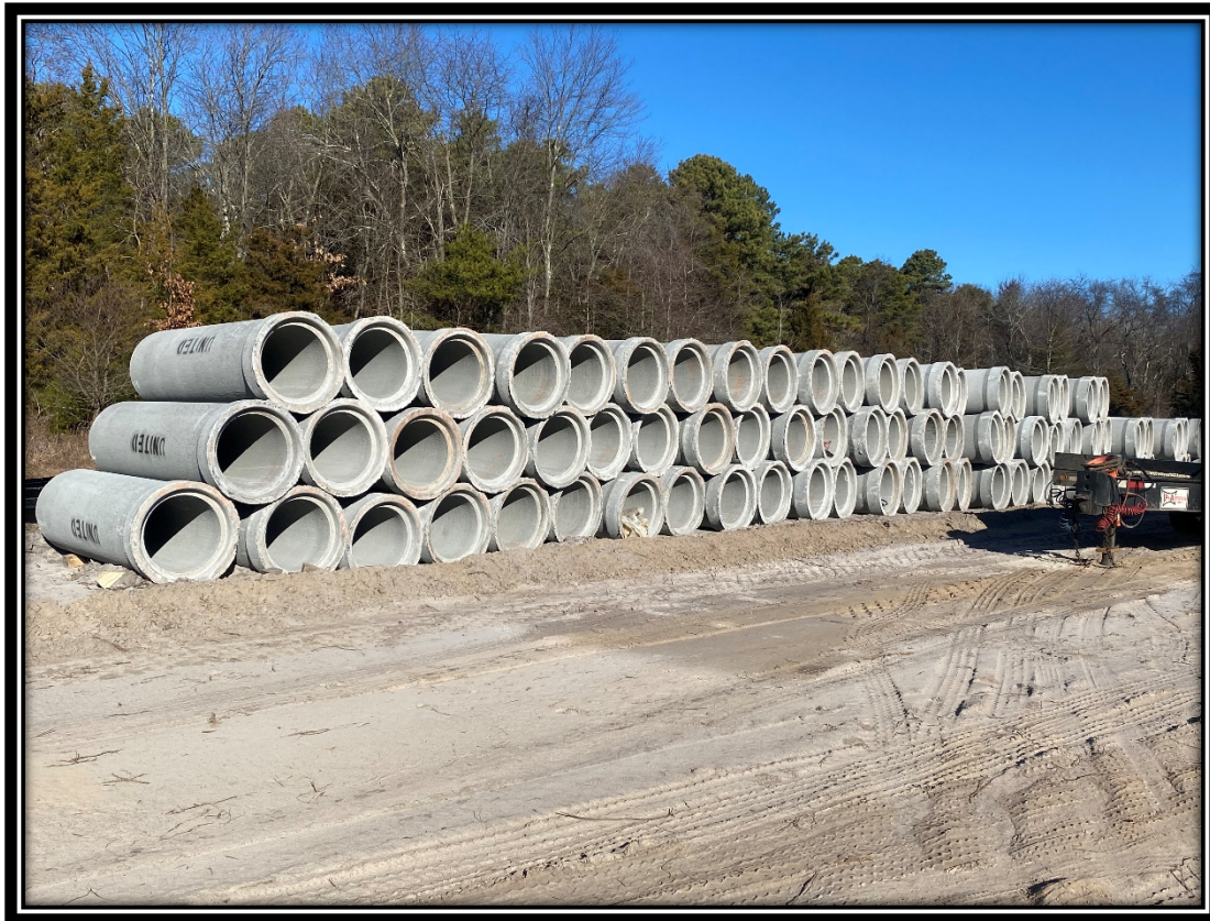
Figure 1: P&A Construction continues to receive reinforced concrete pipe deliveries.
