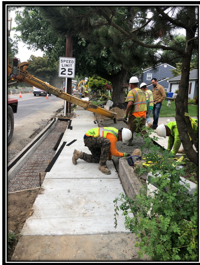
Figure: 1 – Installation of reinforced concrete driveway apron, sidewalk and curb along the westbound lane between Friendship Drive and Millstream Drive
