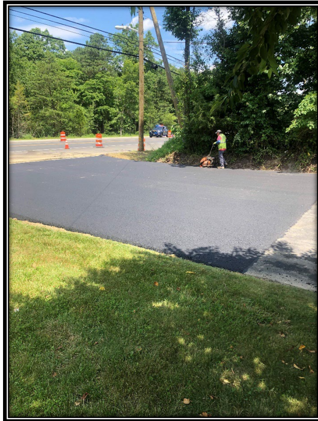
Figure:1 Completed driveway at Albion Church.
