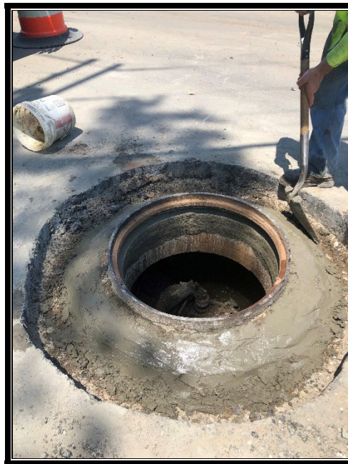
Figure 3: P&A Construction reset manholes in preparation for final paving.
