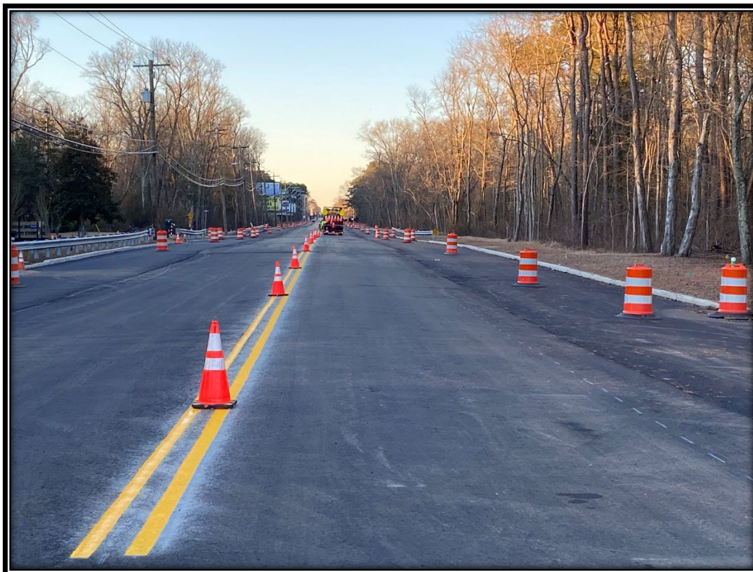
Figure:1 Temporary line striping was completed for the temporary winter shut-down.
