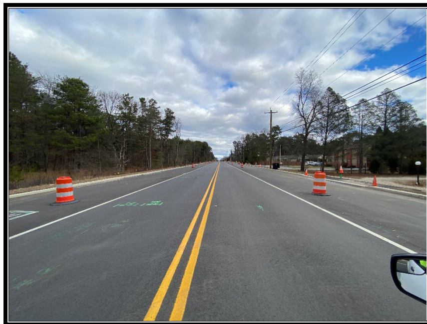
Figure 3: P&A Construction opened two lane traffic on December 20, 2023.
