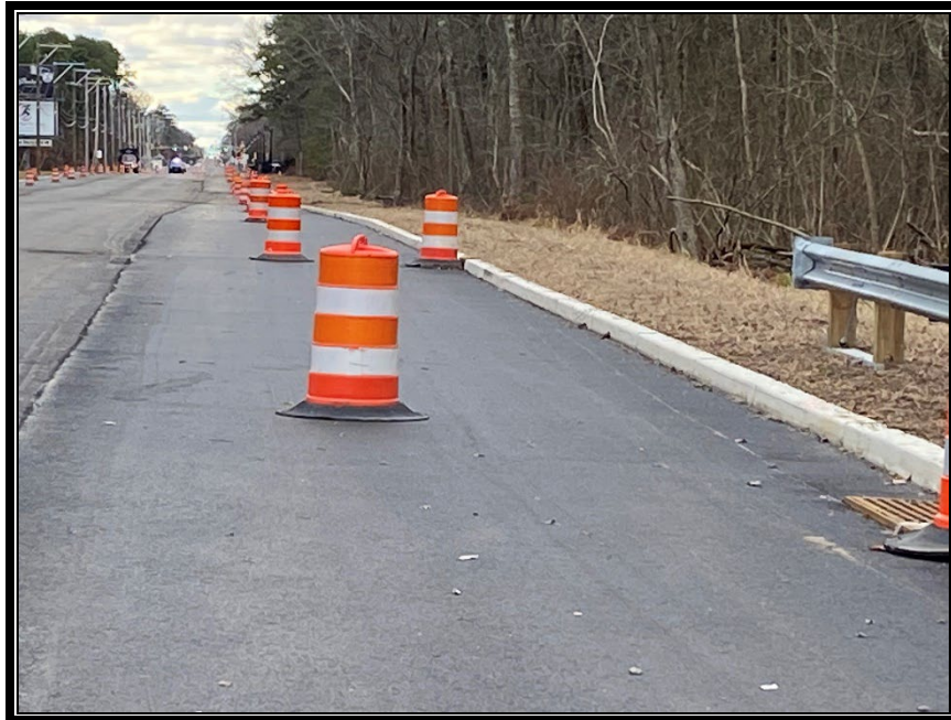
Figure 2: P&A Construction set up temporary traffic control for the winter shutdown.
