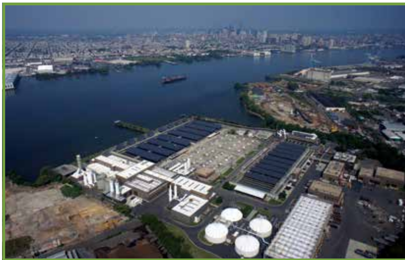
Aerial view of 1.8 megawatt solar array at the Camden County in Municipal Utilities Authority Delaware #1 Facility in Camden, NJ
