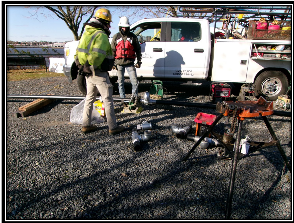
Figure: 2 – Fusing of 3” PVC fire service in preparation for installation
