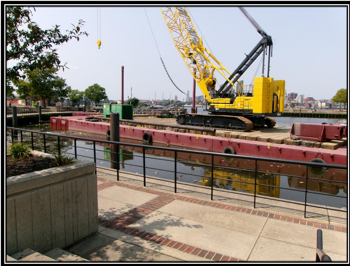
Figure: 1 – Barge and Crane for removal of existing piles
