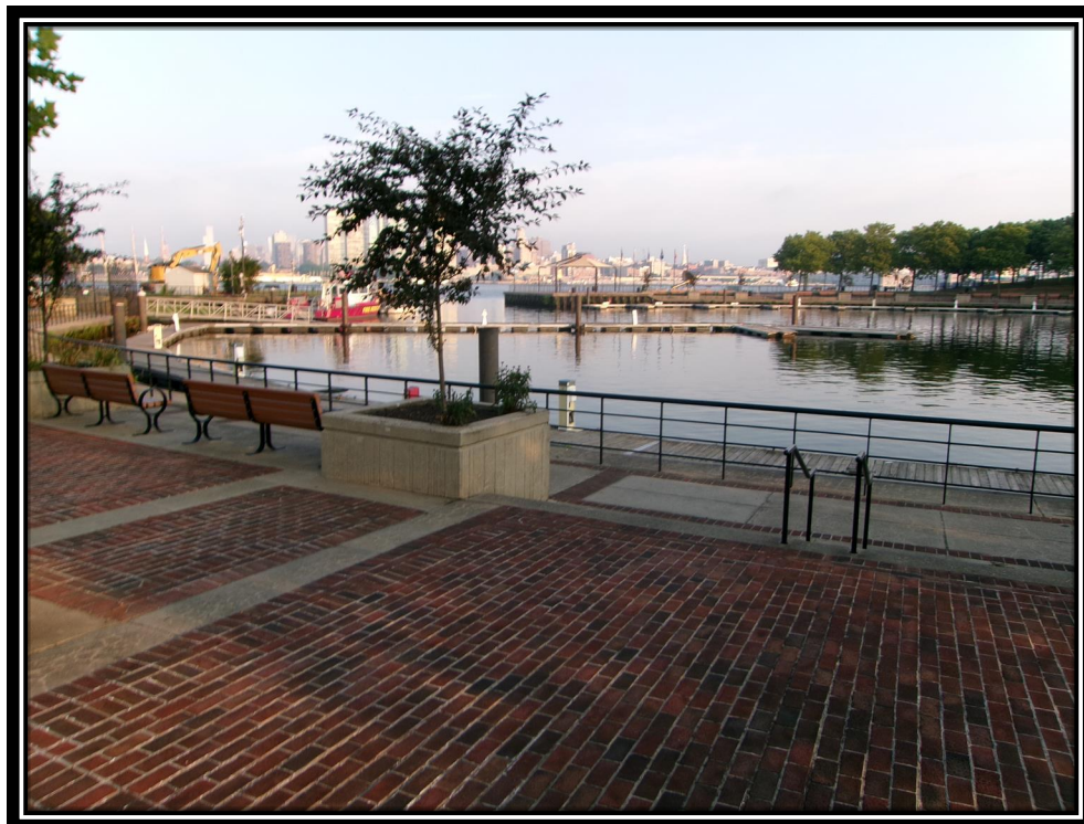
Figure: 3 – Marina after South State removed all of the existing piles as necessary
