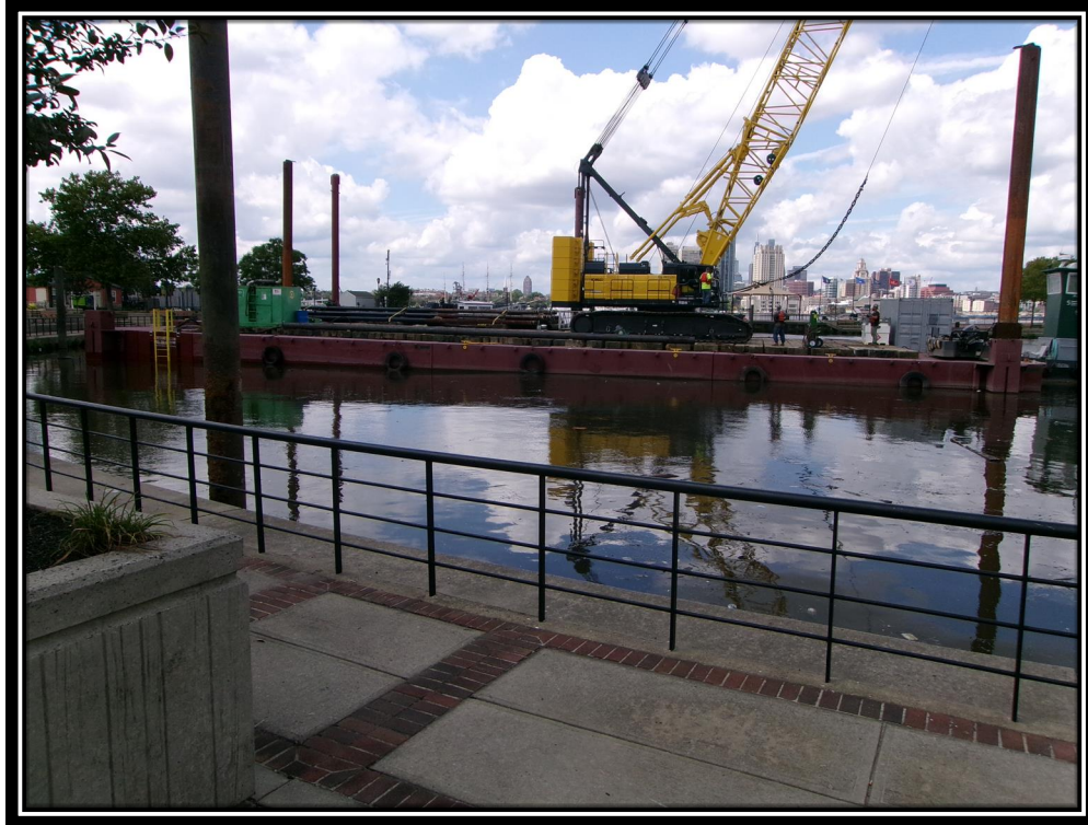
Figure: 2 – Barge and Crane for removal of existing piles
