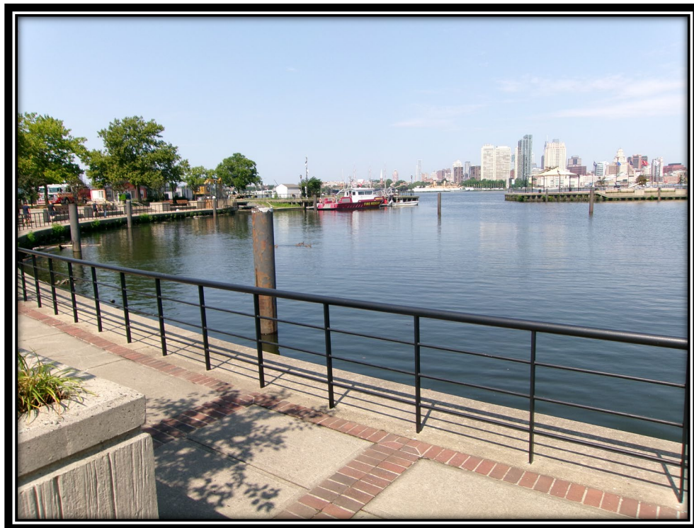
Figure: 3 – Marina after South State removed all of the existing piers and docks
