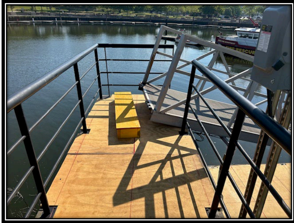
Figure: 2 – Temporary repair of fire dock and gangway
